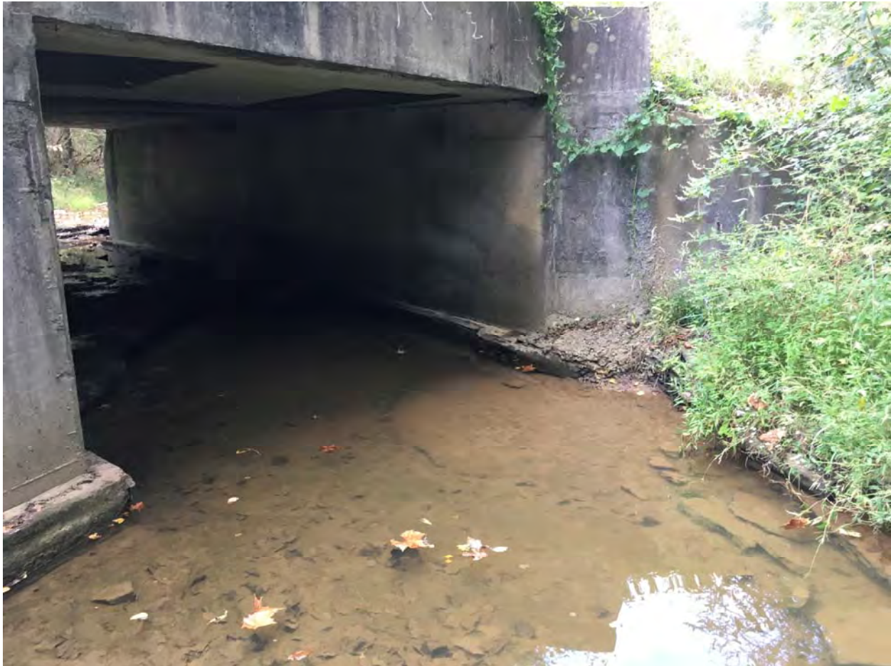
Structure founded on exposed bedrock on KY 2737 @ MP 1.1.
