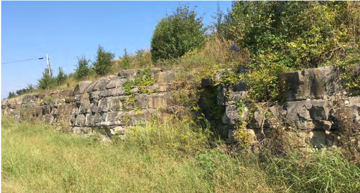
Typical cut slope for dolomite and limestone formations (KY 245 @ MP 6.1-6.2).
